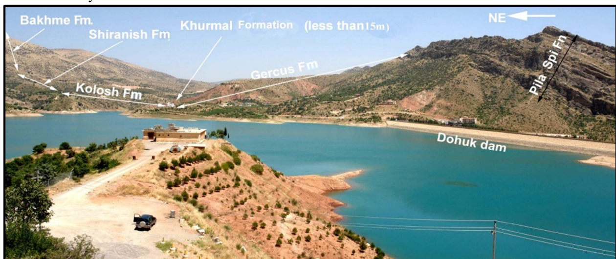
Fig. (4) The eastern part of Duhok dam valley shows outcrops of the formations. The Khurmal Formation is less than 10m thick.
